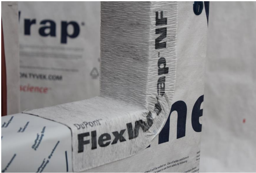
Fig. 9 - DuPont FlexWrap and DuPont Flashing Tape installation.
