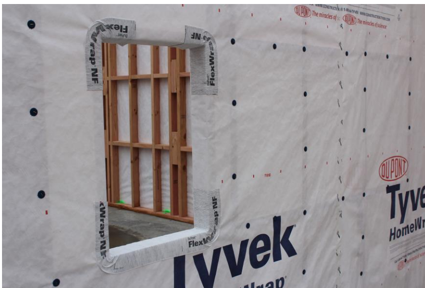
Fig. 10 - DuPont FlexWrap NF only tape installation.
